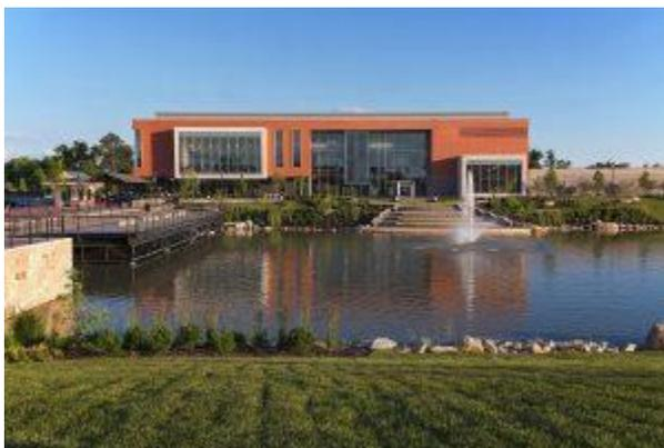
Libbie Mill's landscaping was designed to support stormwater management, incorporates native or adapted plantings, promotes biodiversity and requires no irrigation. The building uses energy-efficient systems and low-flow plumbing fixtures, which are designed to save an estimated 90,000 gallons of water per year. The library's large windows capture natural light and subsequently reduce energy consumption. It also features low-chemical
