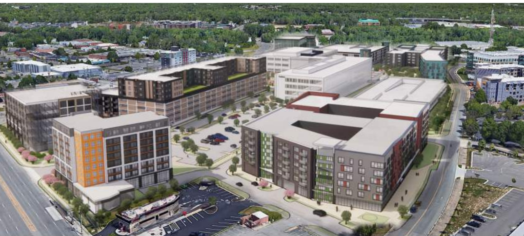
view looking north from Staples Mill Road West Broad Street
