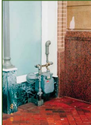
Utilities should not be exposed at the sidewalk because they run the risk of damage.
