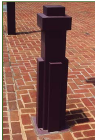
Metal bollards should be treated to resist the deteriorating effects of the elements.
