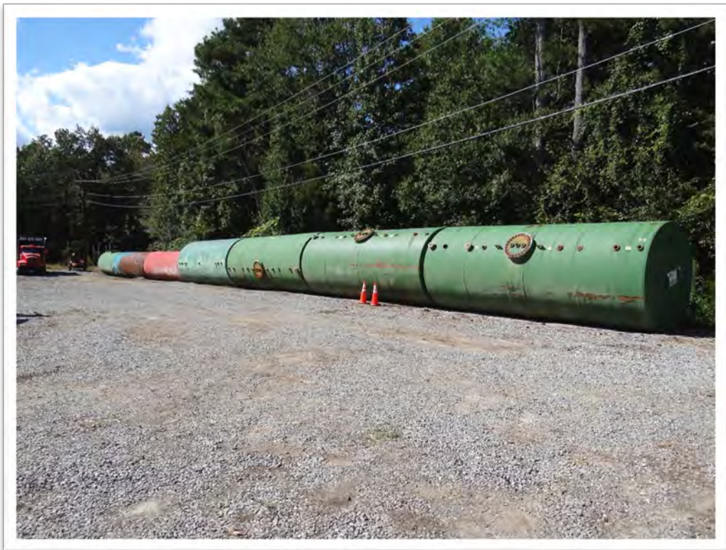
View of tanks along northern property line
