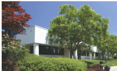
Eastern Government Center 3820 Nine Mile Road 652-3600
