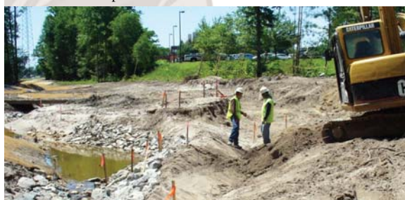
Crews worked to reconnect the Rocky Branch stream to the floodplain and replant native vegetation on its banks as part of a stream restoration project in FY 09.
