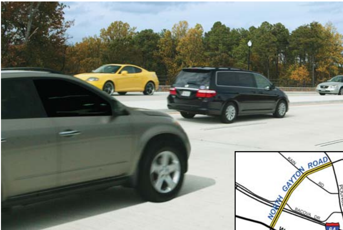
A 2.1-mile extension of North Gayton Road opened Oct. 6 following nearly three years of construction. The $48.4 million project connects North Gayton at West Broad Street to Shady Grove Road at Pouncey Tract Road. The new road, which includes a bridge over Interstate 64, is expected to reduce traffic congestion on Pouncey Tract by providing an additional route to Henrico's northwestern area.
