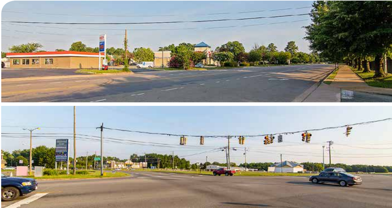
Improvements planned for the Richmond-Henrico Turnpike include new traffic signals, crosswalks and pedestrian signals at its intersection with Azalea Avenue (above), as well as additional traffic lanes, a multi-use path and sidewalks from Laburnum Avenue to the Buckingham Branch railroad crossing (top).
