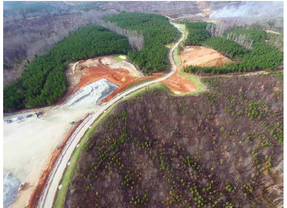
Crews cleared portions of the reservoir site to relocate utility lines.
