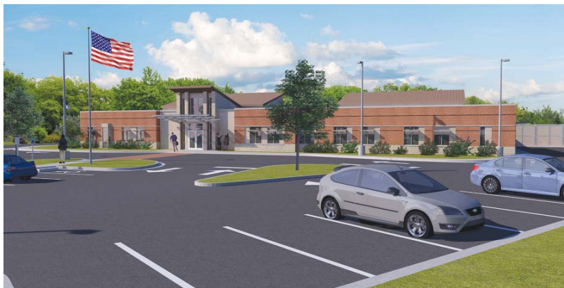
The planned Henrico East Health Clinic will be built along North Laburnum Avenue at Watts Lane. The 13,252-square-foot clinic will provide a larger, permanent space for public health services in eastern Henrico.
