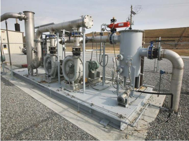
Henrico's Springfield Landfill will soon be the site of an LFG (landfill gas) power plant like this one in New Bern, N.C. The plant will use methane emitted by the landfill's garbage to generate electricity.
