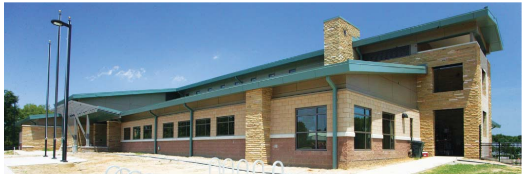
The energy-efficient Eastern Henrico Recreation Center will feature a regulation high school gym, dance studio, walking trails, football complex and other amenities.
