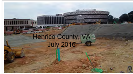
The Faison Residence site, pictured before construction, is near the former Markel building.
