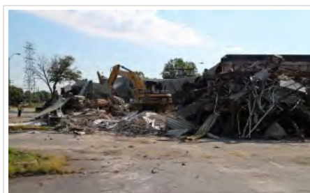
Demolition on some standalone buildings are already well underway.
